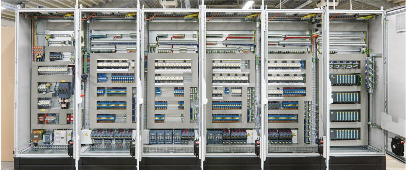
Control cabinets at WAGO are designed with the Cabinet Engineering module from the WSCAD SUITE - including the manufacturing data for the manufacture of the wire sets and cabinet housings on NC machines from well-known manufacturers.
