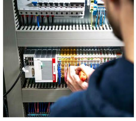
Assembly and wiring of the control cabinets designed with WSCAD are carried out internally at ISAR Aerospace for quality assurance reasons. Source: © Isar Aerospace
